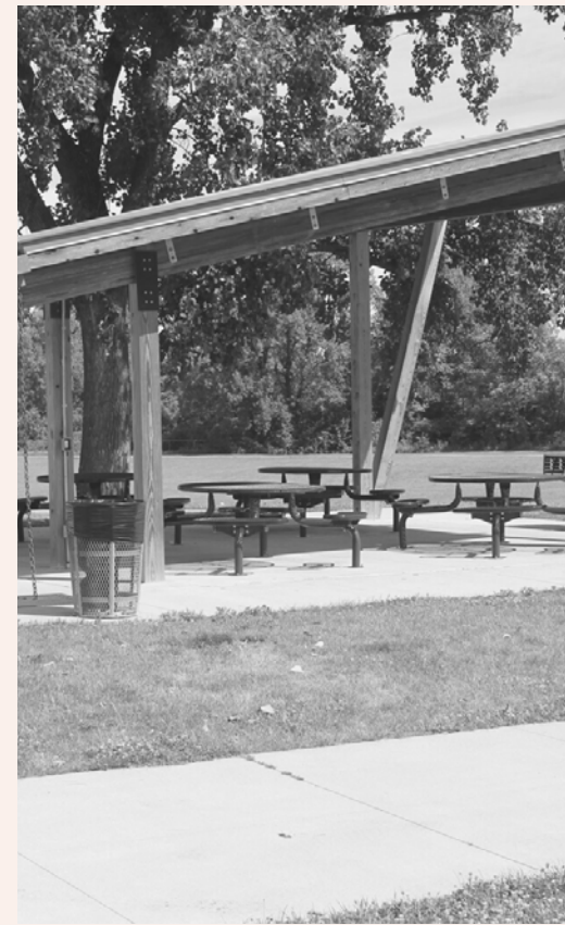
Outdoor Covered Picnic Shelter
