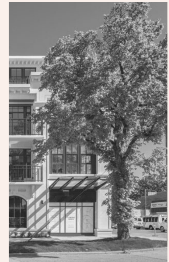
One 3 Storey Building One 4 Storey Building
