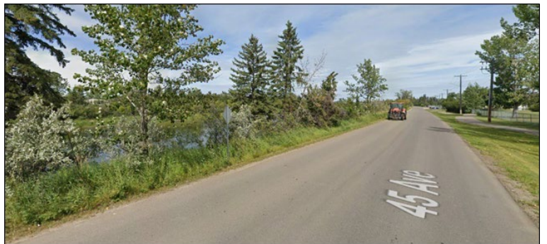
Figure 6 45 Avenue between the river and subject property. Note narrow width of riparian strip, lack of shoulders, lighting, and curbs. (Google Maps 2022)
