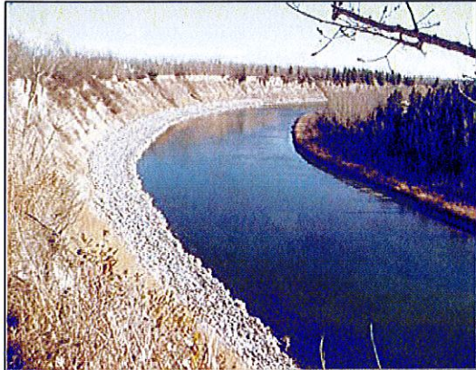
Fig. 10: River Reinforcement at Oriole Park
