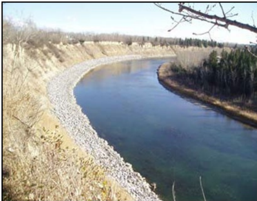
Figure 9 River reinforcement at Oriole Park
