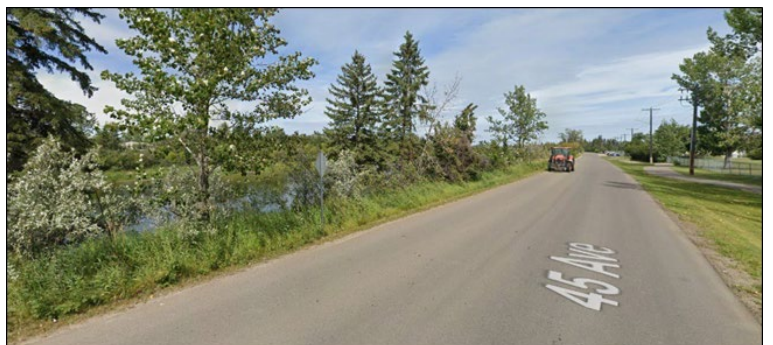
Figure 6 45 Avenue between the river and subject property. Note narrow width of riparian strip, lack of shoulders, lighting, and curbs. (Google Maps 2022)
