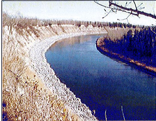
Fig. 10: River Reinforcement at Oriole Park
